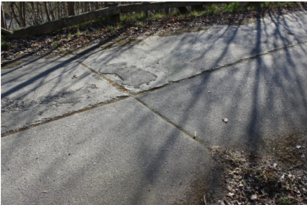
Road surface concrete blocks and their joints.
